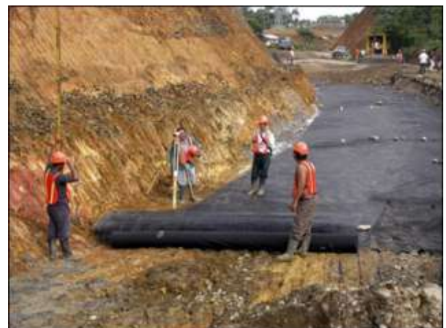
Figure 4: Geomembranes and geosynthetic products to control fluid movement
