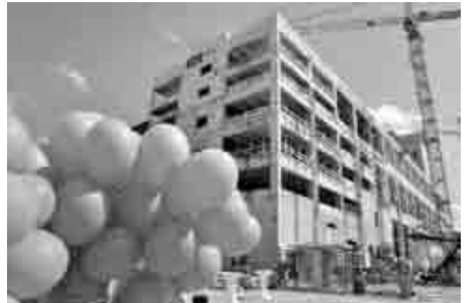
TENCEL® Jumbo line construction Site
