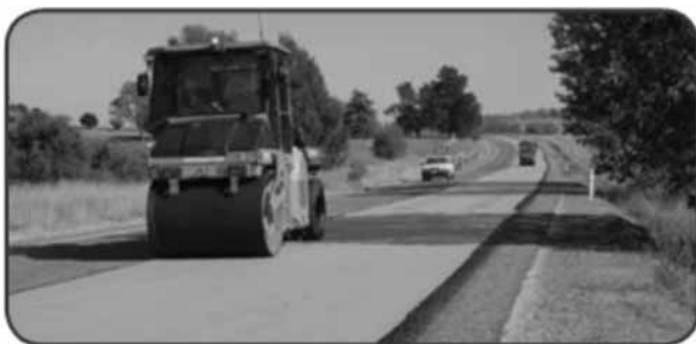
Figure 2.6: Highways and roads construction
