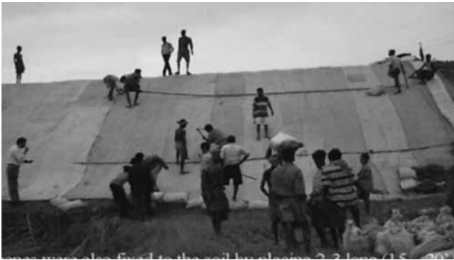
Figure 3.1a: Natural fibre-based geotextiles is being installed on the river bank
