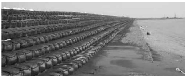
Figure 4.4 : Reclamation bundh at Adani Port
