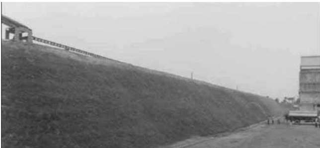
Figure 3.2: Application of erosion control mat (Vishakhapatnam, A.P.)
